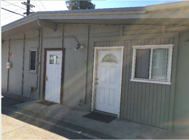
Crew quarters entry
