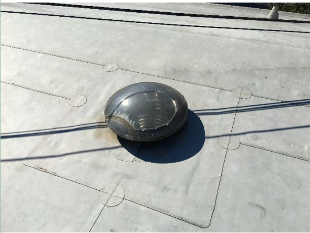
Roof with skylight
