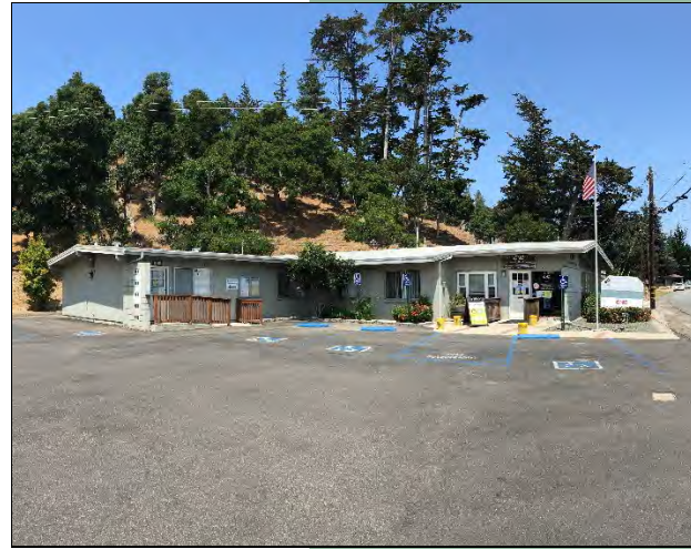
No. of Stories: 1 Square Feet: 3,800
