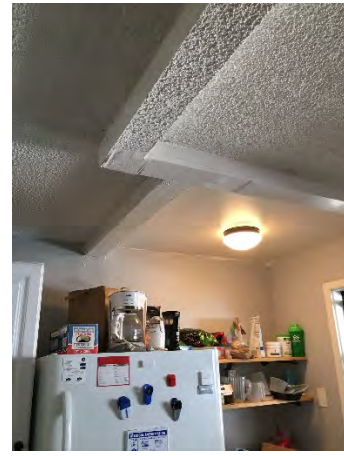
Ceiling at Kitchen
