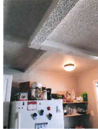
Ceiling at Kitchen
